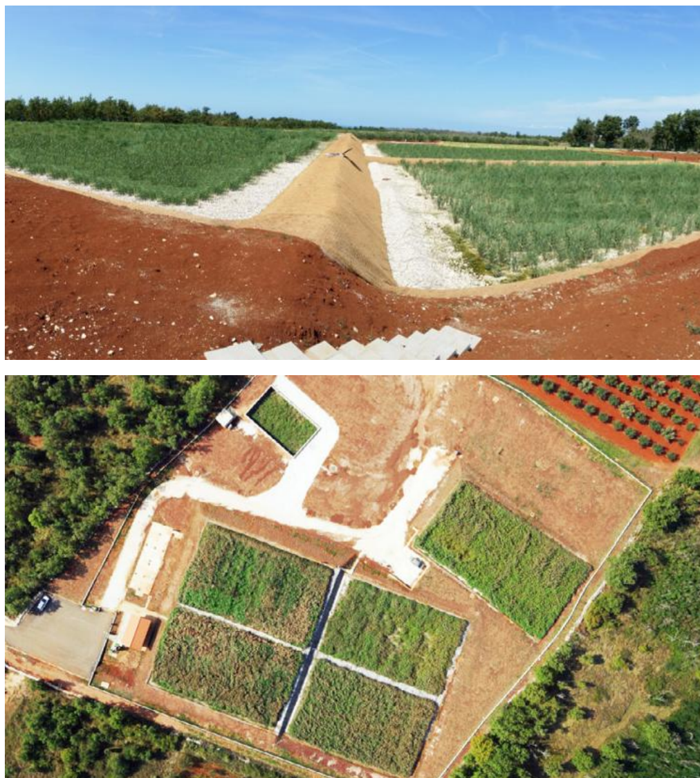
Figure 2-4: Multi-stage Treatment Wetlands system in Croatia – Kastelir treatment plant 2
